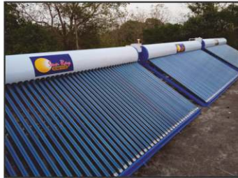
Solar Water Heater
